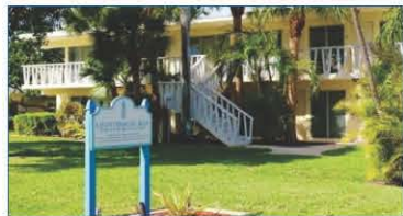
MARINA AREA -5LIGHTHOUSE PT. $235,000.
